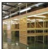
**Structural Mezzanine Floors** leave a large open area below for maximum working space. This can be utilised for various different uses i.e. office area, packing area, storage area or receiving or dispatch area.
